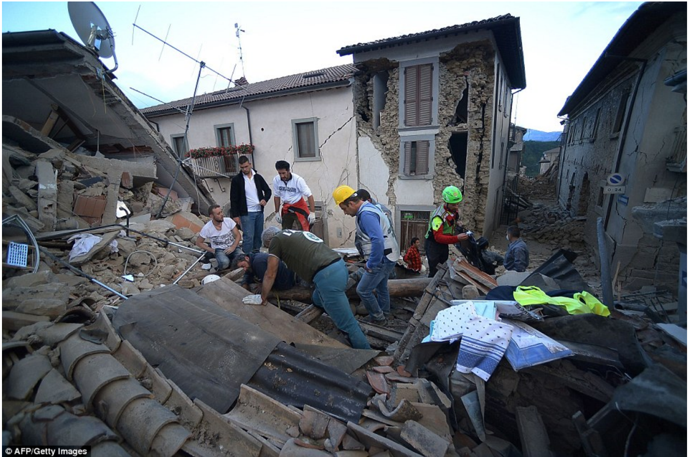
Desperate: This is all that is left of a building in Amatrice where emergency services and volunteers pull away tiles and rubble searching for victims
