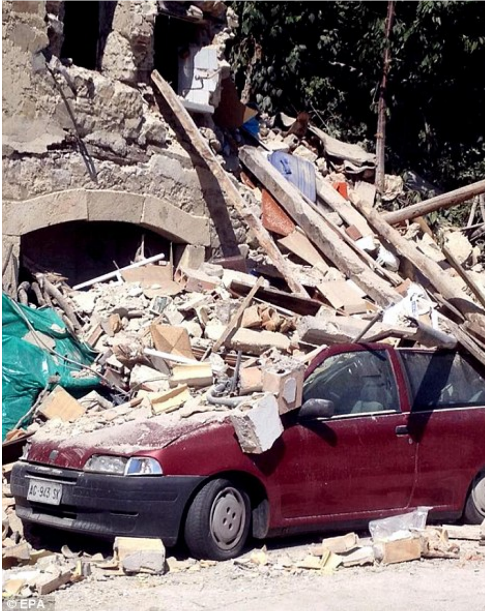
Impaled: A concrete post smashed through a car windscreen (left) in the Reatino area on Wednesday and another car (right) was buried in Pescara del Tronto
