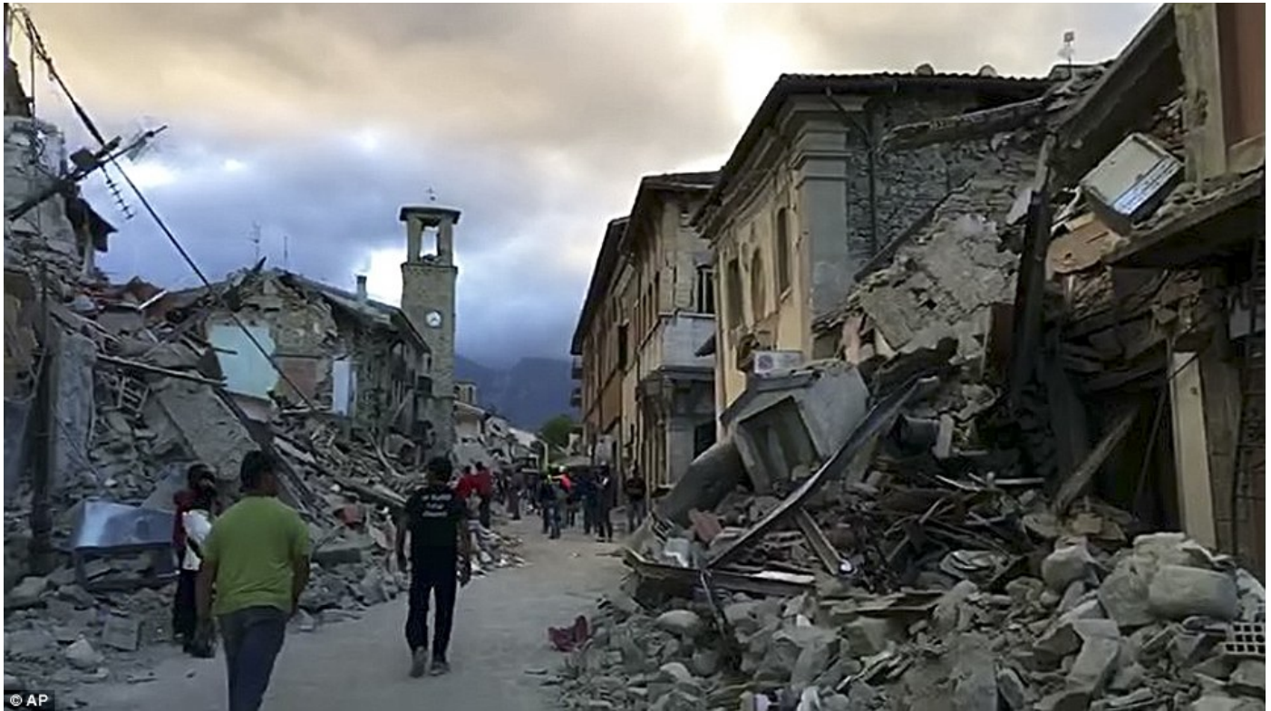
Aftermath: Residents of Amatrice in central Italy has been left in ruins overnight in an earthquake that shook areas up to 100 miles away, including Rome
