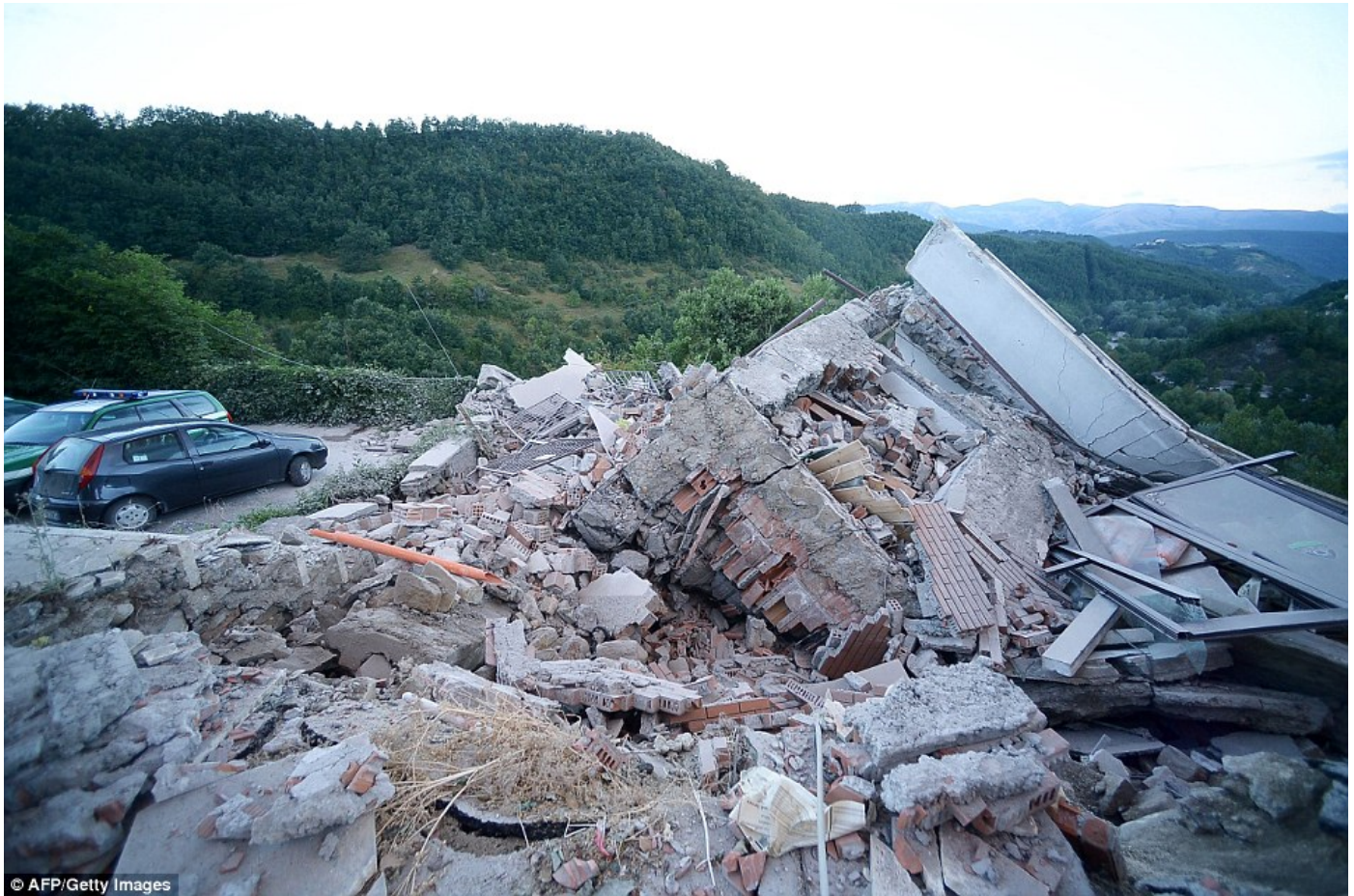
Many buildings in center of Amatrice were razed by the 6.1 magnitude quake, which struck at around 3.30am (local time)
