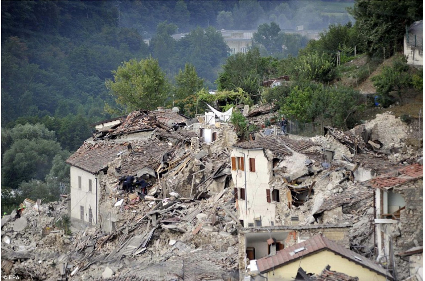
Collapsed houses are seen crumbling down the mountain side in Pescara del Tronto, near Arquata del Tronto municipality
