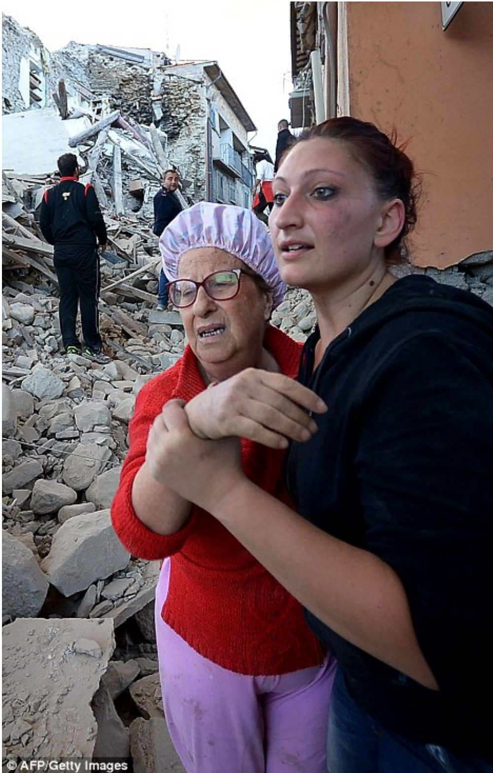
The devastating earthquake tore down entire streets and homes in Amatrice (pictured), close to the epicenter of the quake in central Italy
